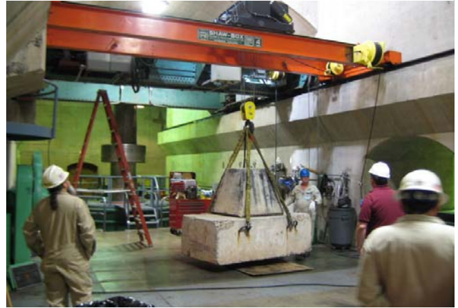
Load Testing—New 5 Ton Capacity, ACT Trolley
