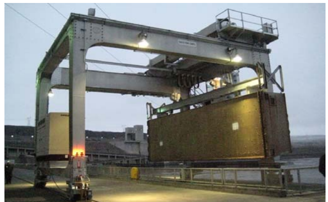
Rehabilitated 50 Ton Tailrace Crane at Lower Monumental Dam
